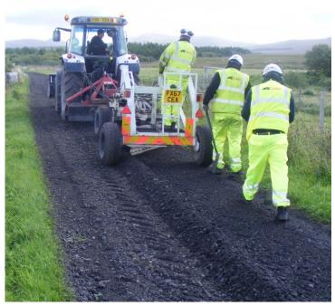
The photo below shows part of the surface dressing process which is a preventative treatment aimed at sealing the road surface from the ingress of water whilst restoring surface texture to worn or slippy surfacing. The treatment enables surfacing service life to be extended by 5-10 years prior to a more robust resurfacing project being undertaken to strengthen and reshape the carriageway.
